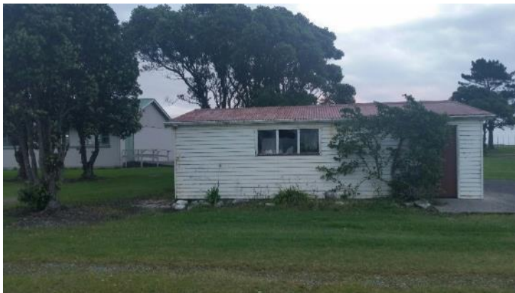
Figure 4-3: Old shed near community facilities on Carters Beach domain reserve. [Credit: P. Birchfield, 10/05/2017].
