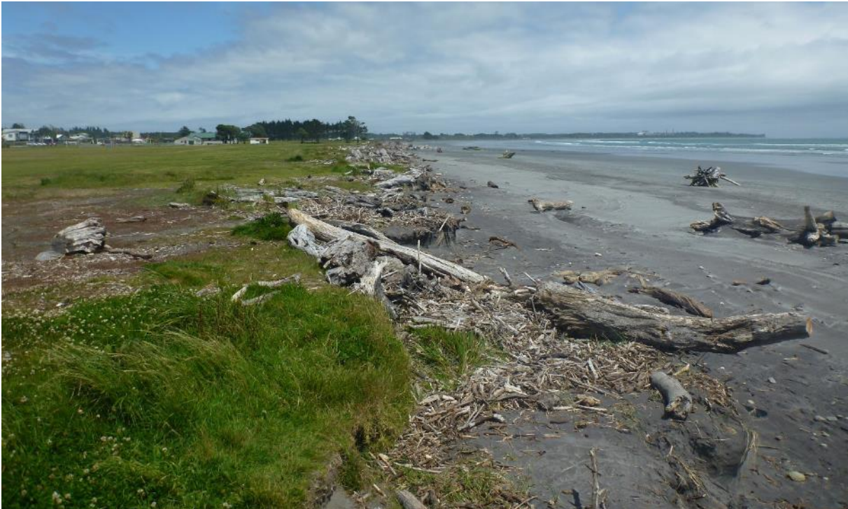
Figure 2-3: Evidence of coastal retreat at Carters Beach foreshore. Accessed at Golf Links Road. [Credit: M. Hicks, 23/11/2016].
