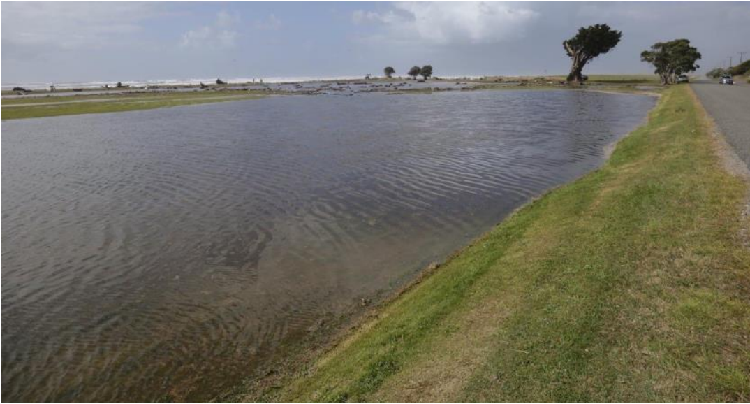
Figure 2-6: Sea water ponding in the Carters Beach domain reserve after 16 January 2017 wave overtopping event. Note Marine Parade at right. [Credit: C. Cooper, 16/01/2017].
